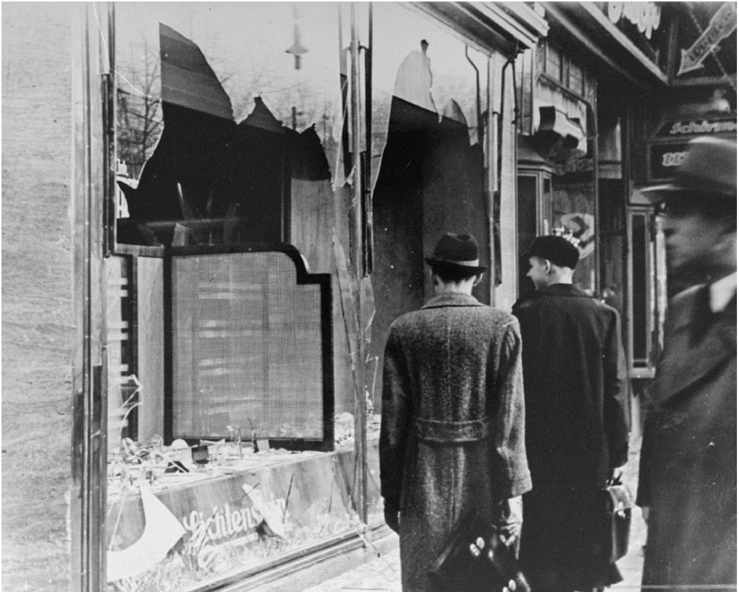
Windows of a store that was damaged during Kristallnacht
